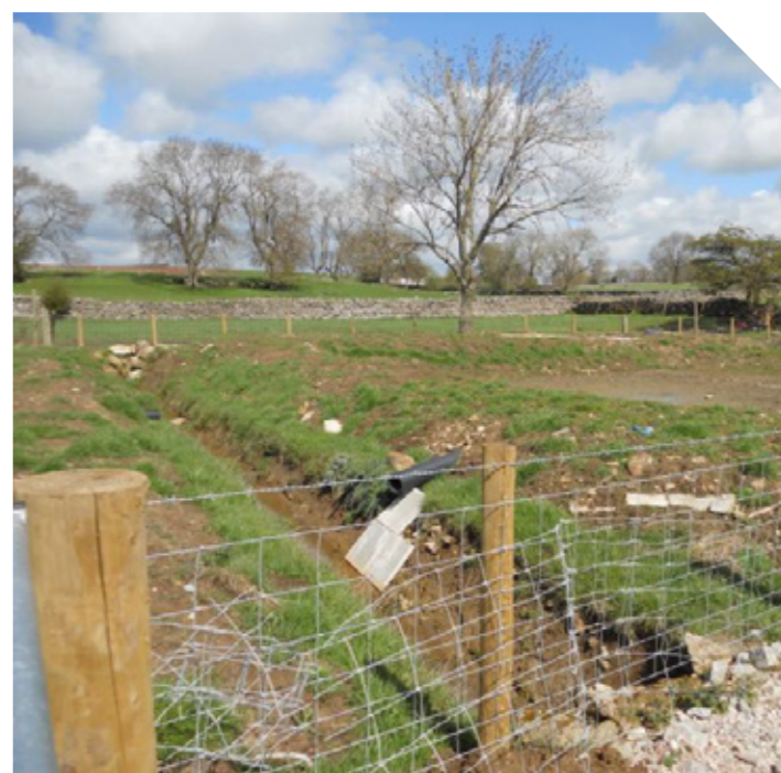
OVERLAND FLOW INTERCEPTION VIA IN-FIELD DETENTION POND AT A TENANT FARM IN LOWTHER ESTATE, MORLAND CATCHMENT
