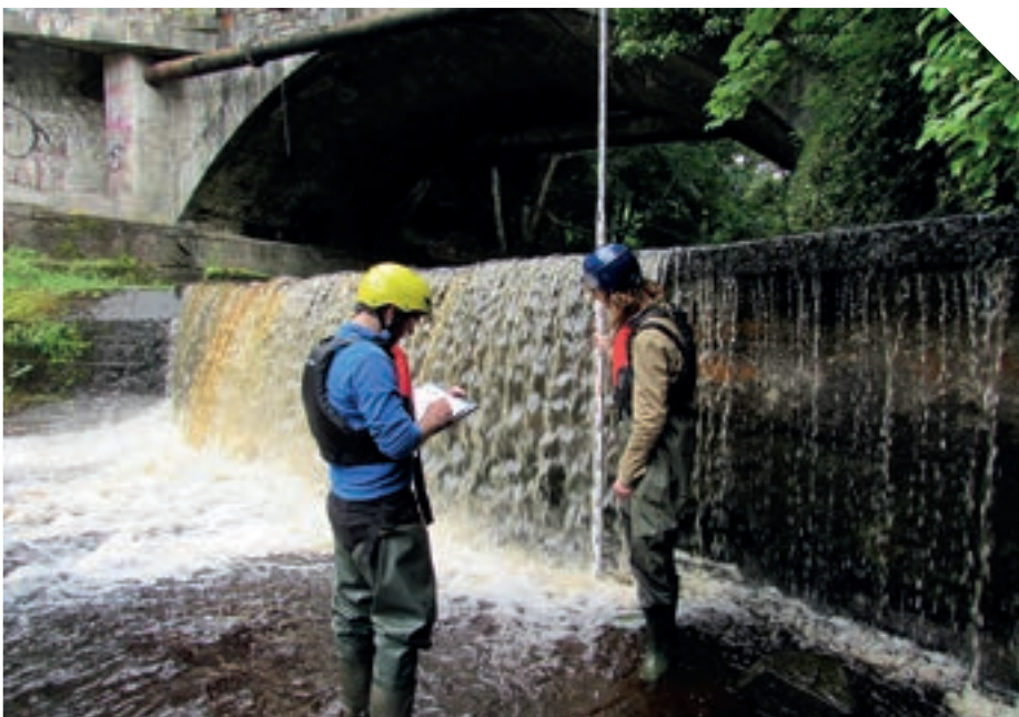
SURVEY OF A BRIDGE APRON ON THE RIVER DODDER
