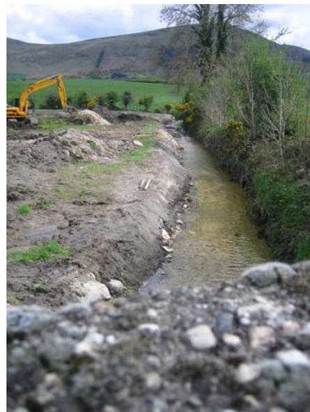
**Plate 3.9 & 3.10 Bank alteration works within the Ballymurphy Catchment**
