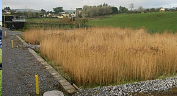
Sludge Drying Reed Beds
