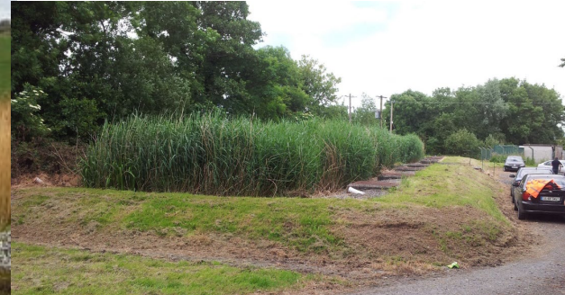
Reedbeds Polishing Filter
