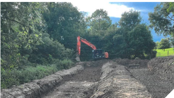
Levelling and compacting the sides and base for planting of reeds and multispecies grasses. Soil with higher clay content introduced to seal the base.
