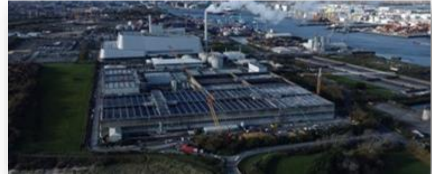
Ringsend Wastewater Treatment Plant upgrade - €500m (ongoing)
