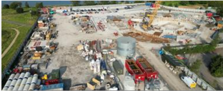
Athlone main drainage scheme €114m (wastewater)
