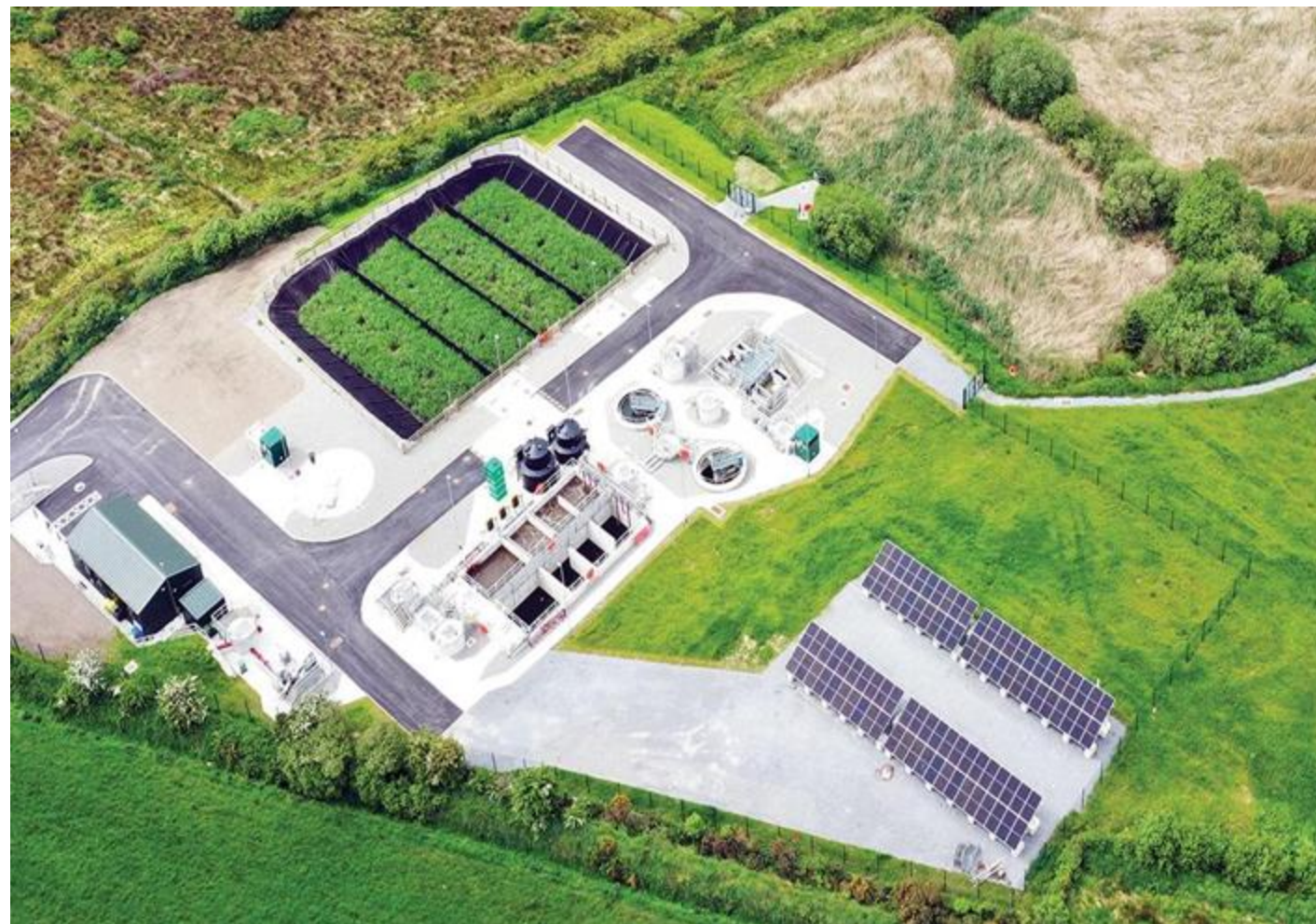
Boherbue WWTP March 2026
