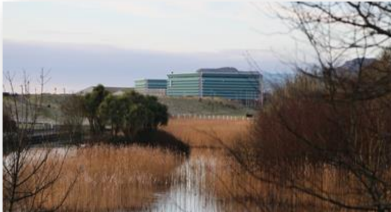
Arklow Wastewater Treatment Plant upgrade - €139m (complete)
