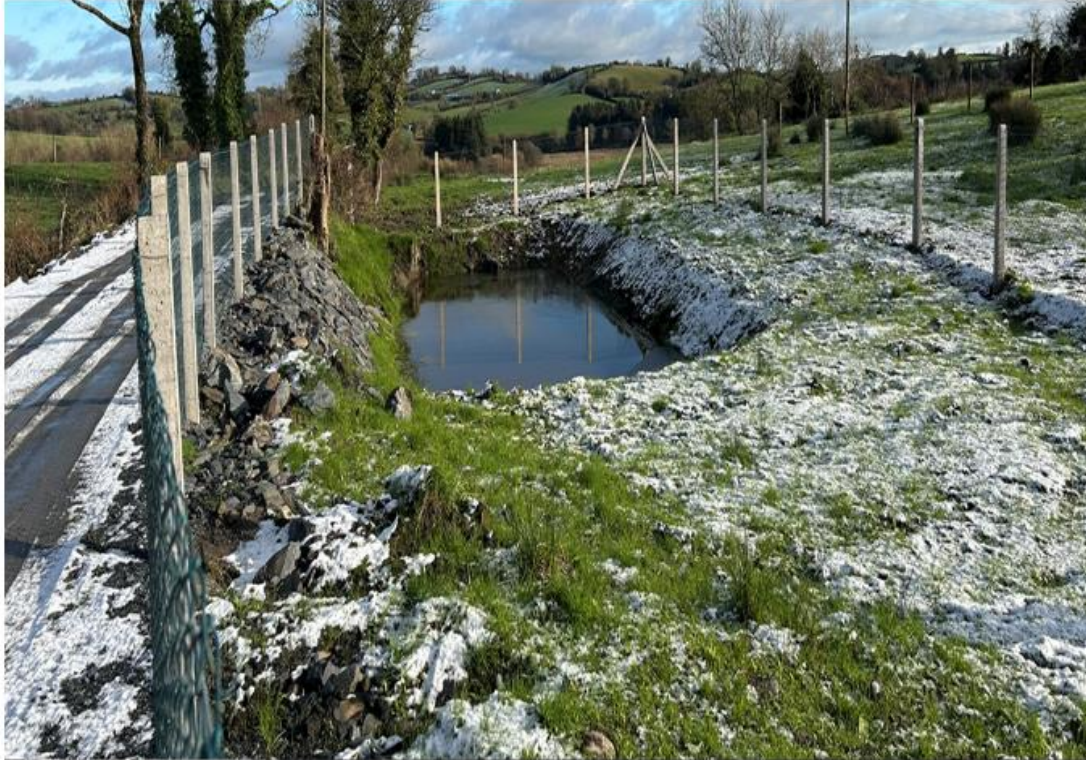
Newly constructed Pond
