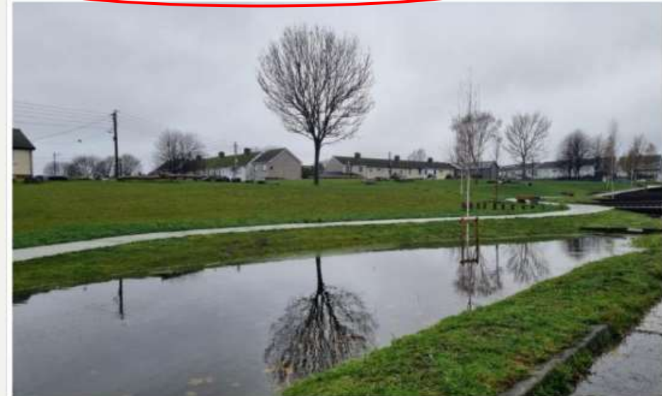
The Rainscapes Project at Lein Road, Artane – showing short-term stormwater retention post storm event.
