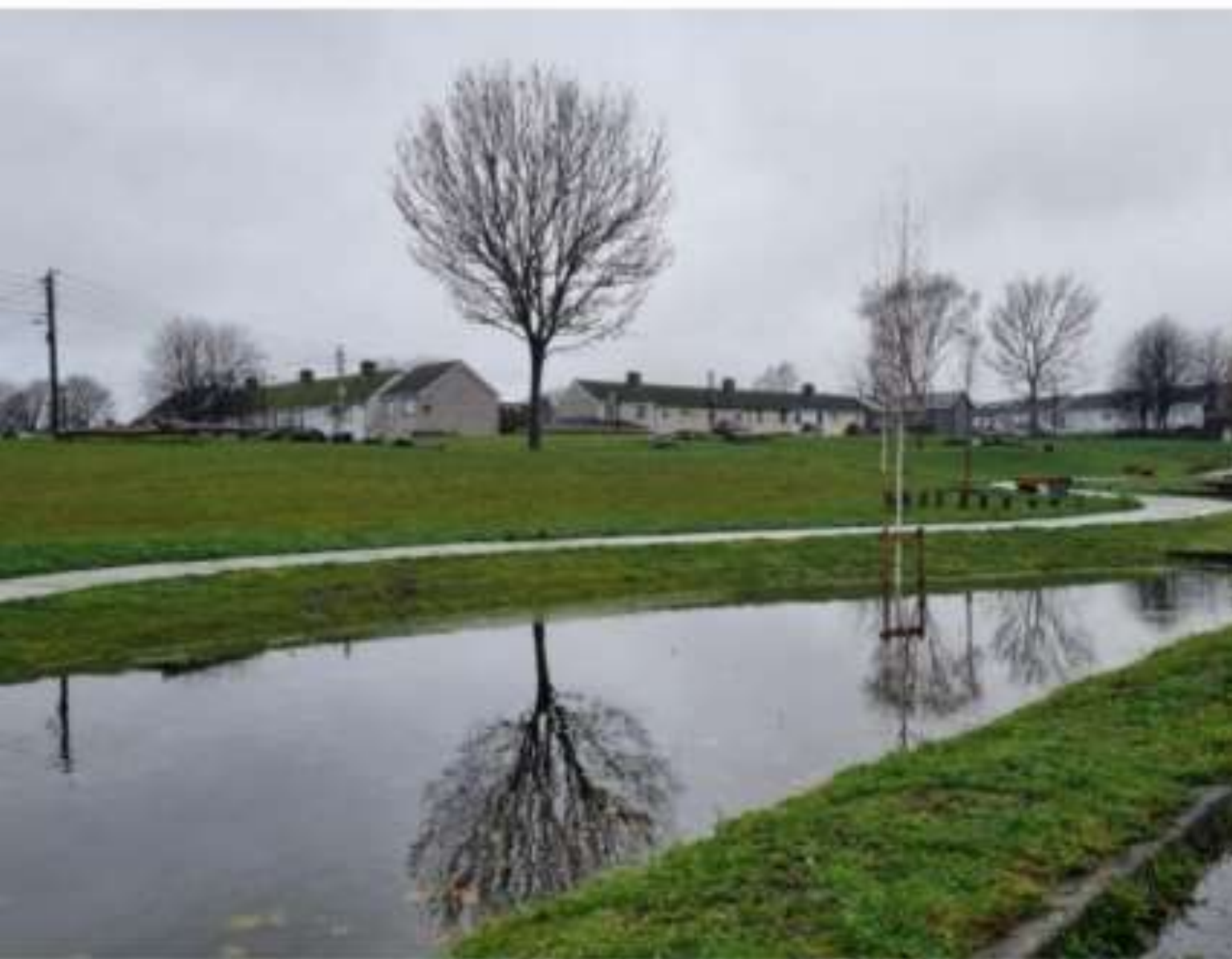
Rainscapes Project at Lein Road, Artane – showing short-term stormwater retention post storm event.
